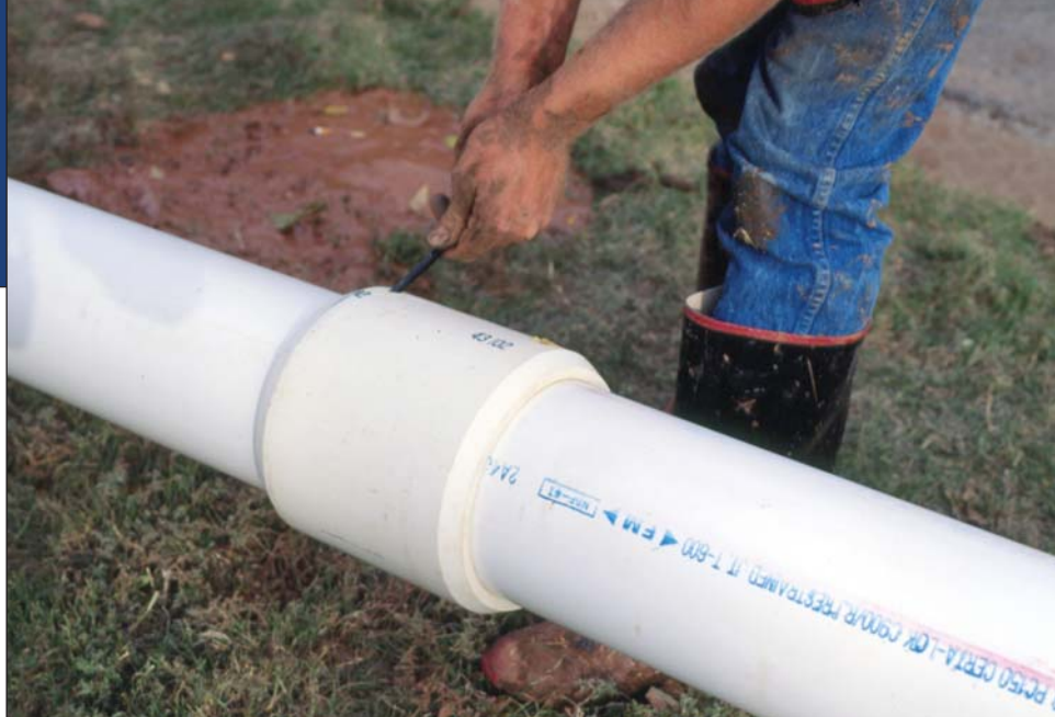
Restrained joints lock lengths of pipe firmly together and can be made as fast as lengths of drill pipe are removed from the drill string, making it unnecessary to assemble a long string of pipe for installation.
